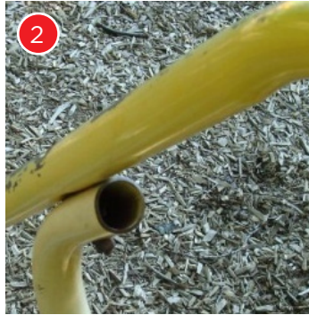
The cap is missing and should be replaced.
