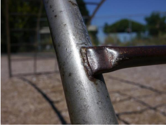
No welded joints are broken, rusting, or rough
