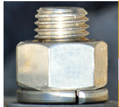
Check that bold ends show less than 2 threads and are rounded and smooth
